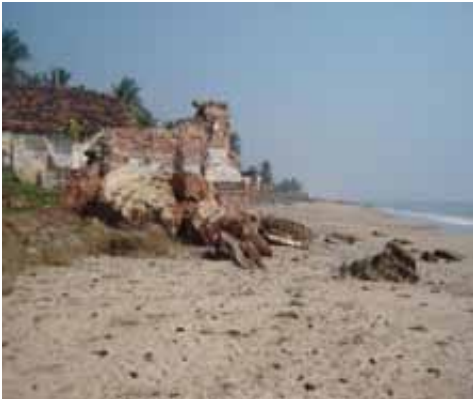
Temple collapsed near Uppada
